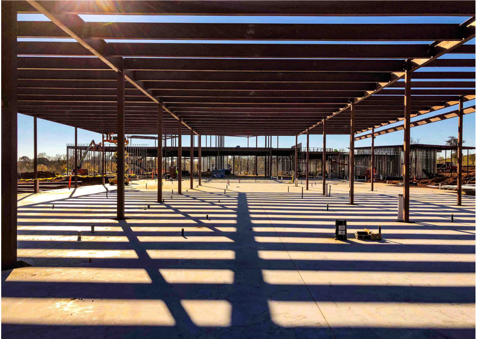
Construction Site Beams
